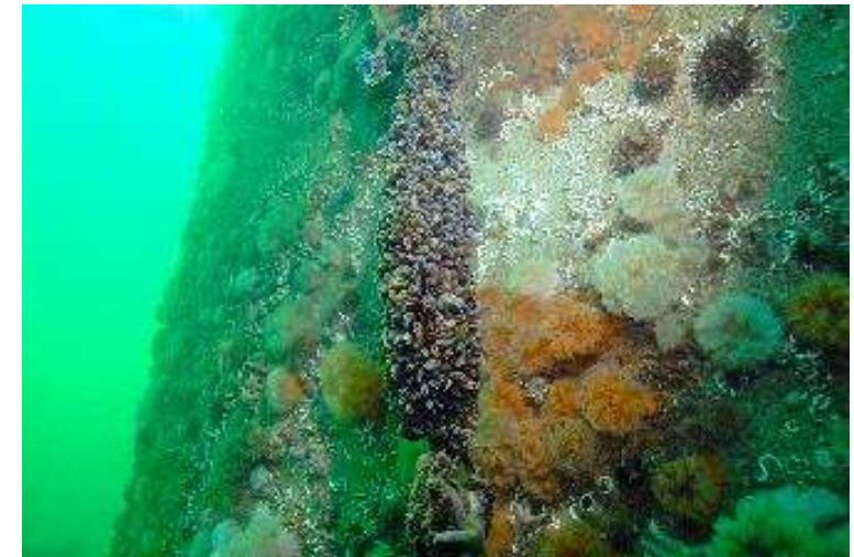
Concrete offshore gravity-based wind turbine foundation, blue mussels, plumose anemones, sea urchins, common starfish, barnacles, and tubeworms. Photo credit: Royal Belgian Institute of Natural Sciences, Alain Norro.
